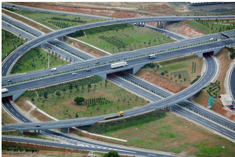
Western Egaleo Peripheral Interchange
