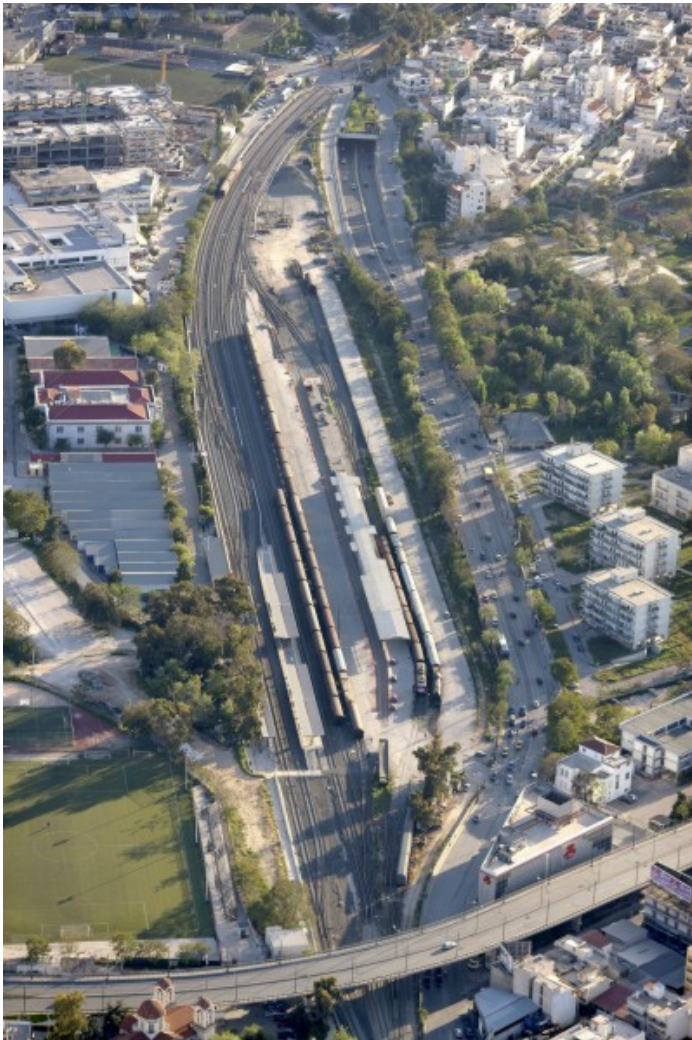
“Roof” cargo station and stabling yard
