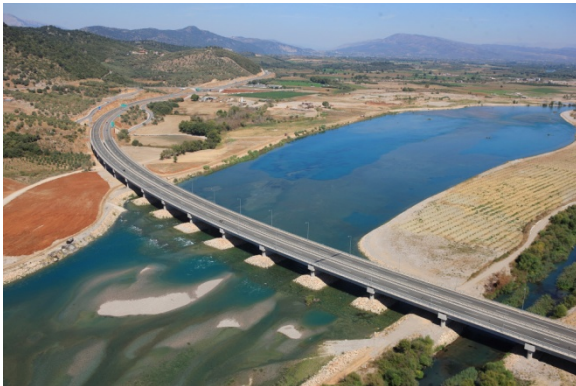
Ionia Odos Motorway, Greece. Acheloos crossing.
