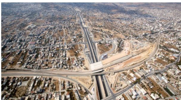
SKA Multimode Transfer Facility, north-west view, Greece
