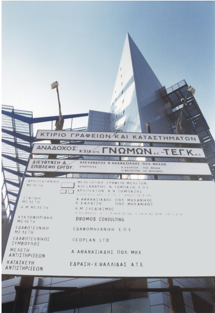
Office building, Mavrakakis property, Greece, with two underground parking levels.
