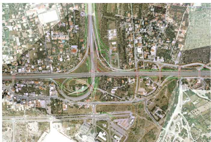
Korinthos to Patras Motorway, Greece. Reconfiguration of Rio interchange
