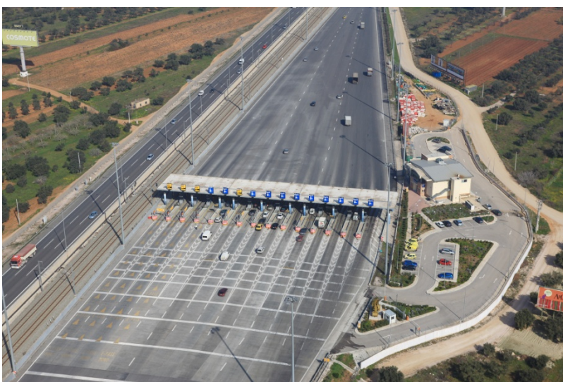
Koropi frontal toll plaza
