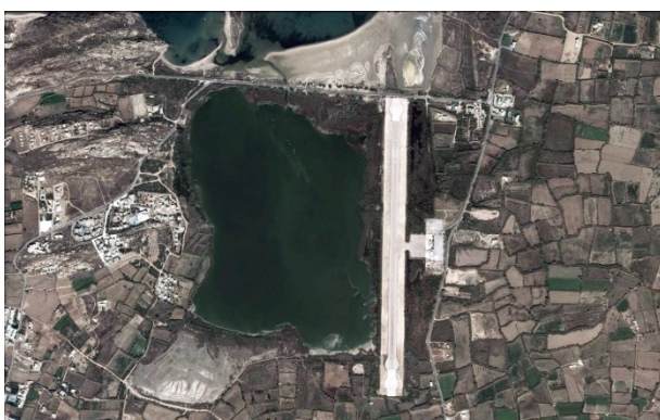
Naxos island New Airport, Greece.
