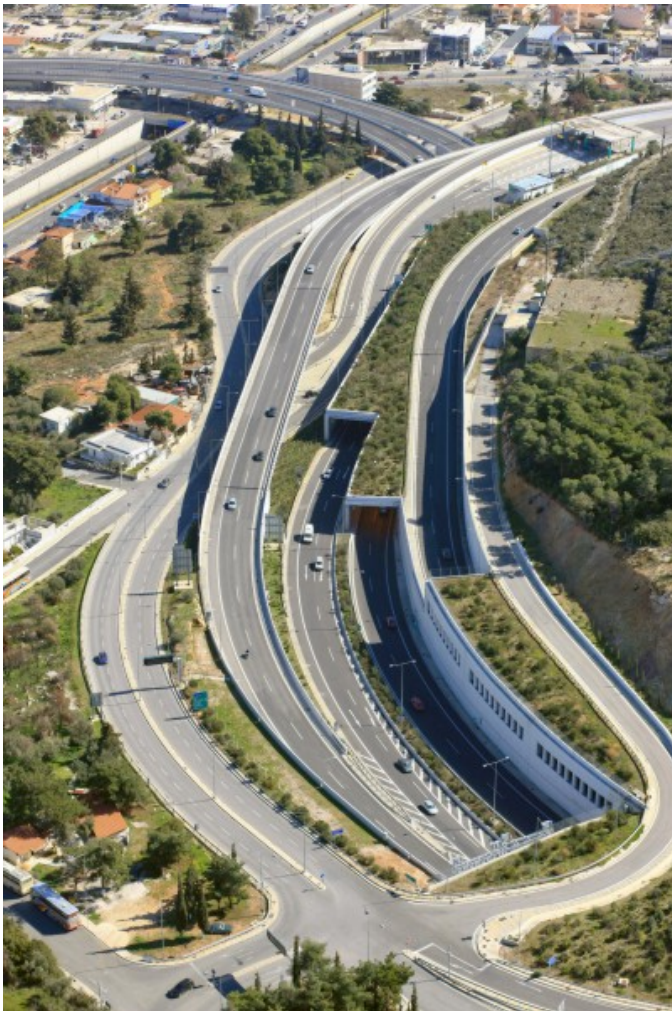
Ag. Paraskevi interchange
