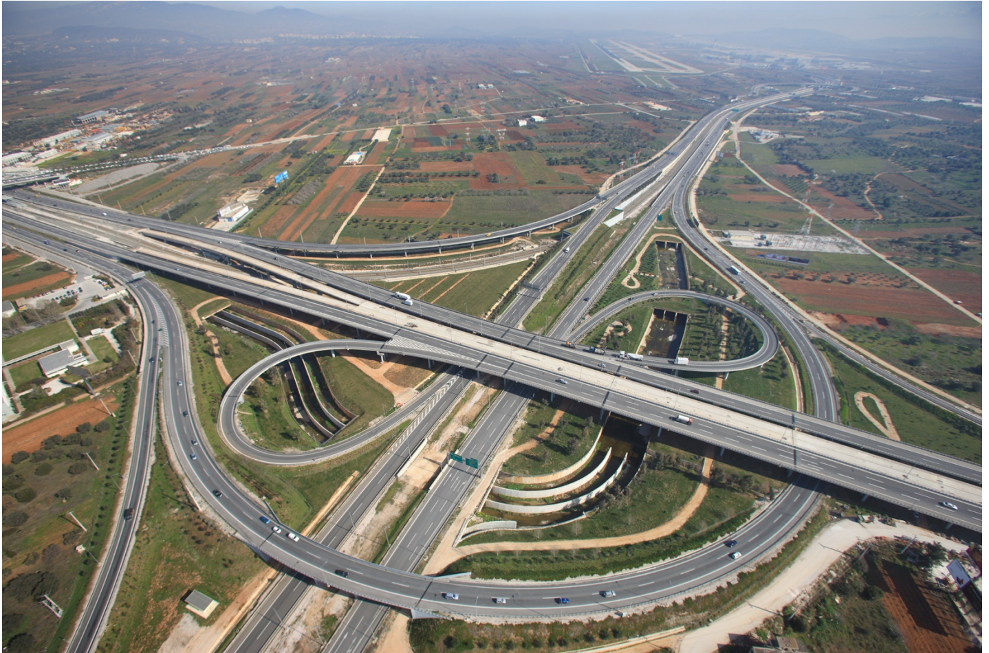
New Airport interchange
