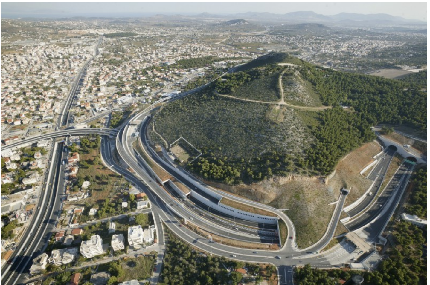
Western Imittos Peripheral branching interchange
