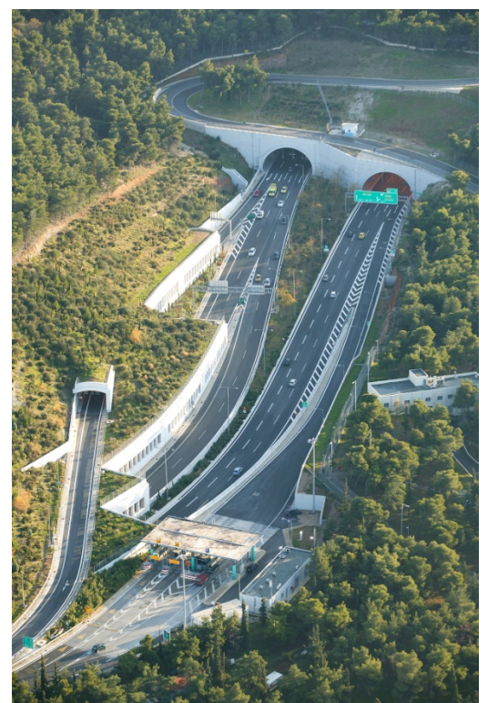
Ag. Paraskevi interchange
